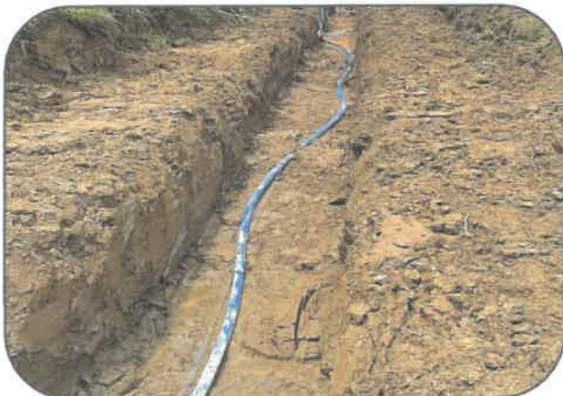
New PVC waterline on West Berkshire Road
