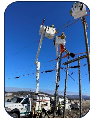
Crews conducting line work
