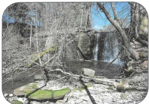
Trout Brook Dam slated for removal
