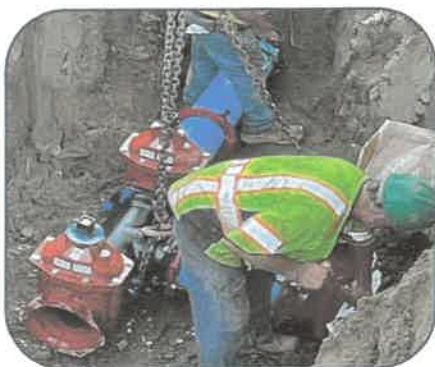
New Waterline being Installed by Munson Earth Moving
